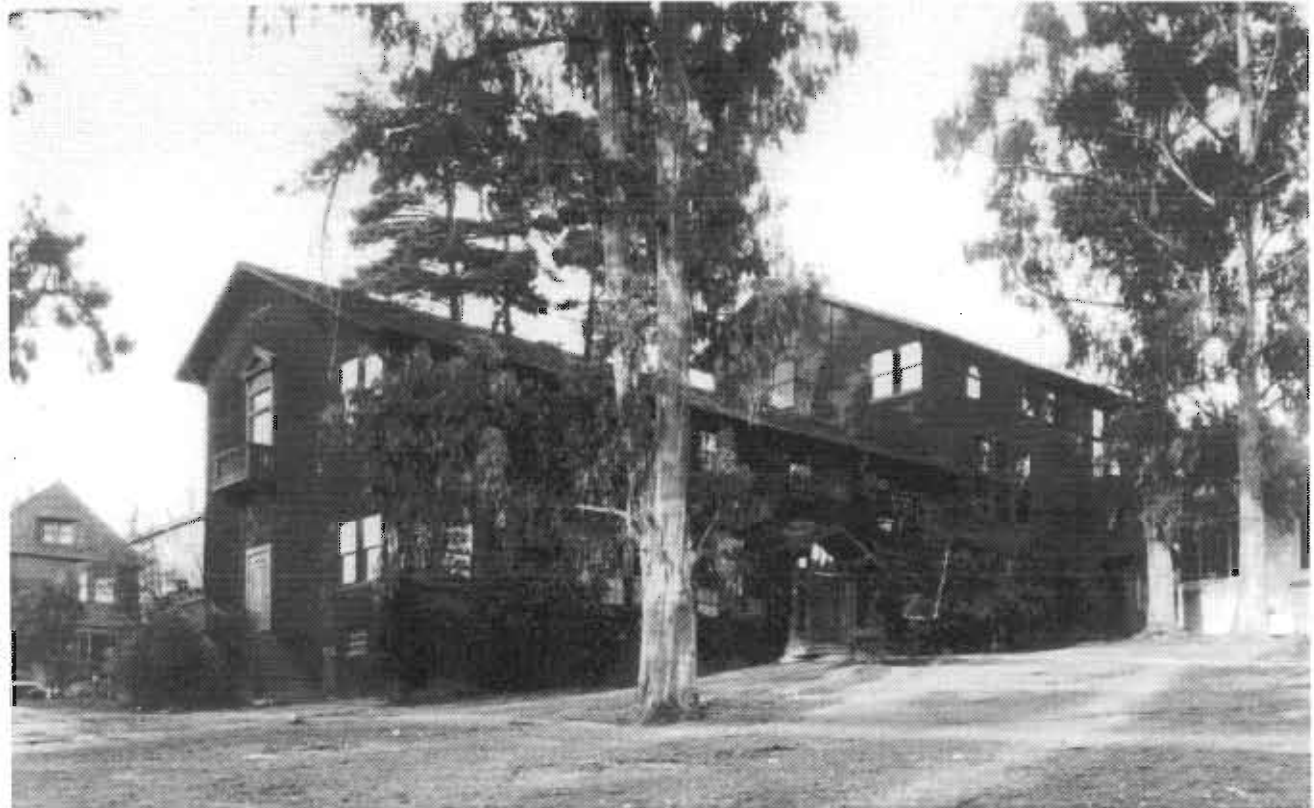
Figure 9. After demolition of the eastern half of the Addition (+/- 1932)
