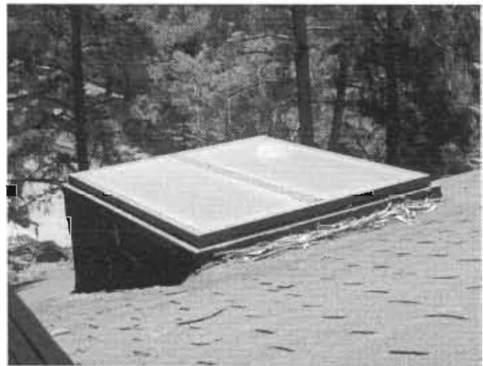
Figure 23. Skylight at Room #203
