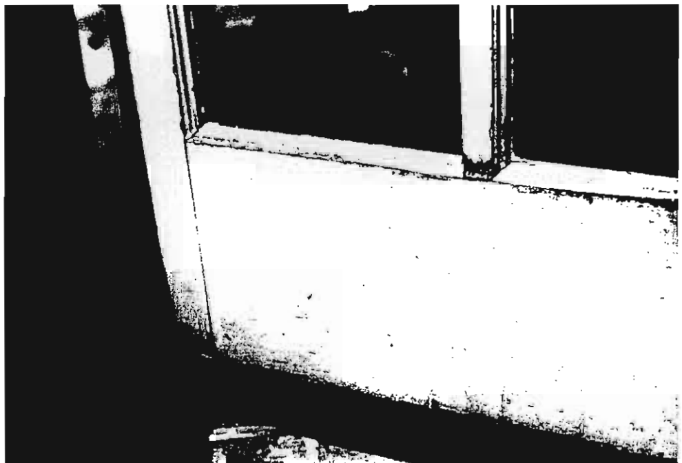
2e. Glazing and sash conditions: Balcony door sash.
