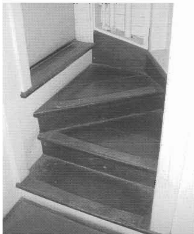
Figure 31. Winding stair to Room #203
