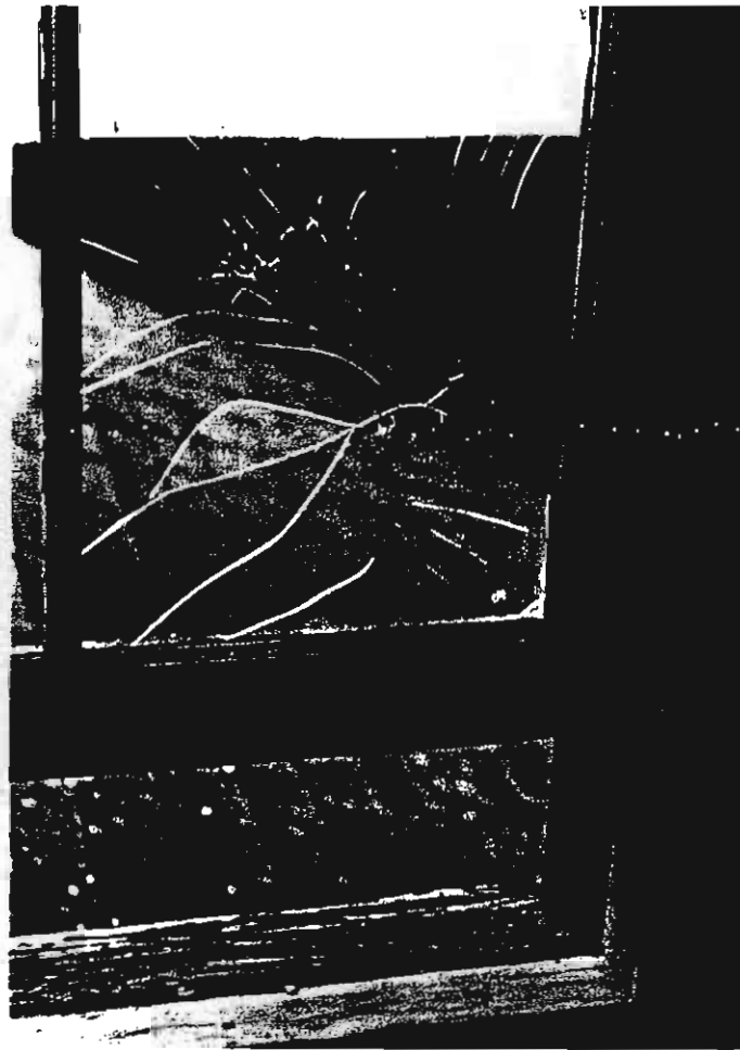
2d. Glazing and sash conditions: Broken window pane, rotted sill at 3rd floor classroom.
