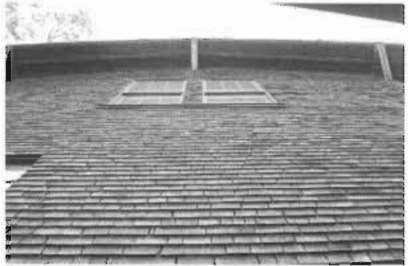
Figure 20. East Facade showing windows at Room #300
